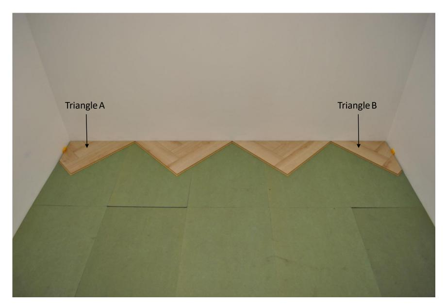
Install the first Left Planks (marked "Gauche" = G) with the Black Plastic tongue pointing to the left
