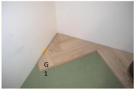
Installing the Right Planks (marked Droit = D)
