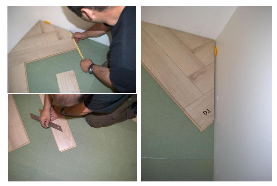
Measure and fit the piece G2 (from Left Plank)
