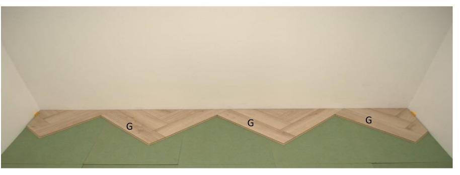
Next install the missing Left Plank piece G1
