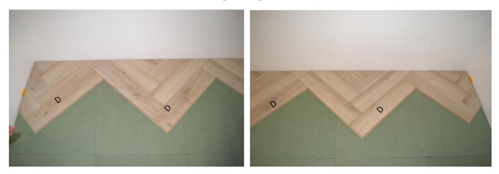
Measure the missing Right Plank piece D1
